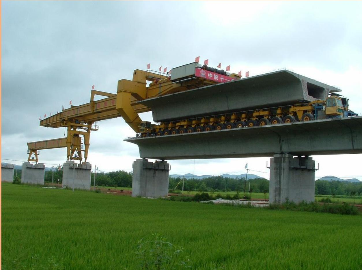
The SLJ900/32, made by the Beijing Wowjoint Machinery Company, is a 580 ton, 300 foot long and 24 foot wide mega machine that looks more like a train than a crane. Instead of using a stationary or crawler crane to lift the girder of a bridge from the ground and drop it into its place, the SLJ900/32 drives the girder onto the previously placed girder, slowly extends its arms to the next support platform, pushes the girder towards the front of the machine and then lowers it into place.
