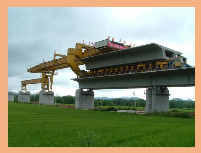
The SLJ900/32, made by the Beijing Wowjoint Machinery Company, is a 580 ton, 300 foot long and 24 foot wide mega machine that looks more like a train than a crane Instead of using a stationary or crawler crane to lift the girder of a bridge from the ground and drop it into its place, the SLJ900/32 drives the girder onto the previously placed girder, slowly extends its arms to the next support platform, pushes the girder towards the front of the machine and then lowers it into place.
